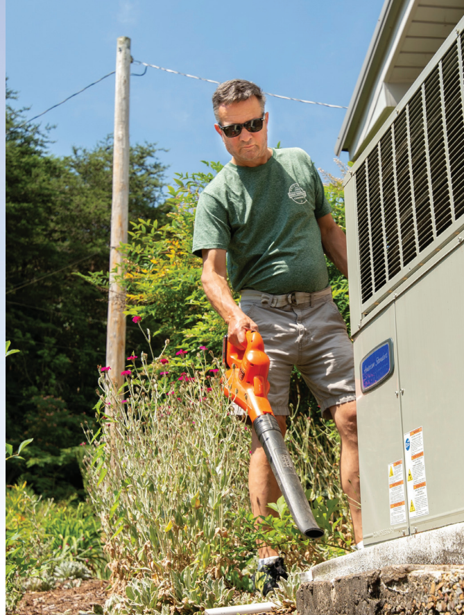
Offer to clean up leaves and debris around your neighbor's air conditioner or heat pump. This will keep the system running efficiently. PHOTO BY MARK GILLILAND/PIONEER UTILITY RESOURCES
